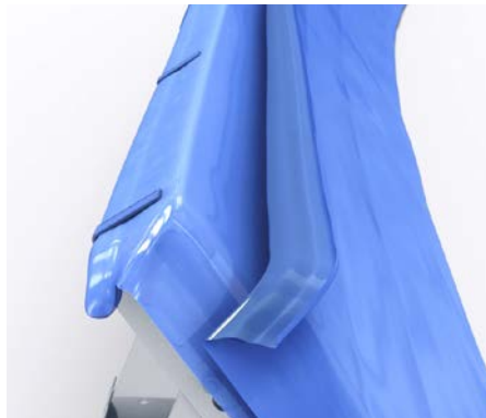
5. Fix the membrane with clips
